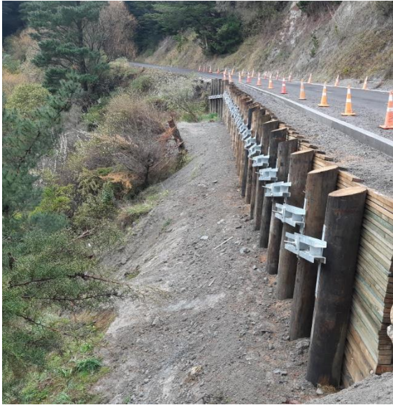
Ormondville Te Uri Tie back wall prior to sealing
