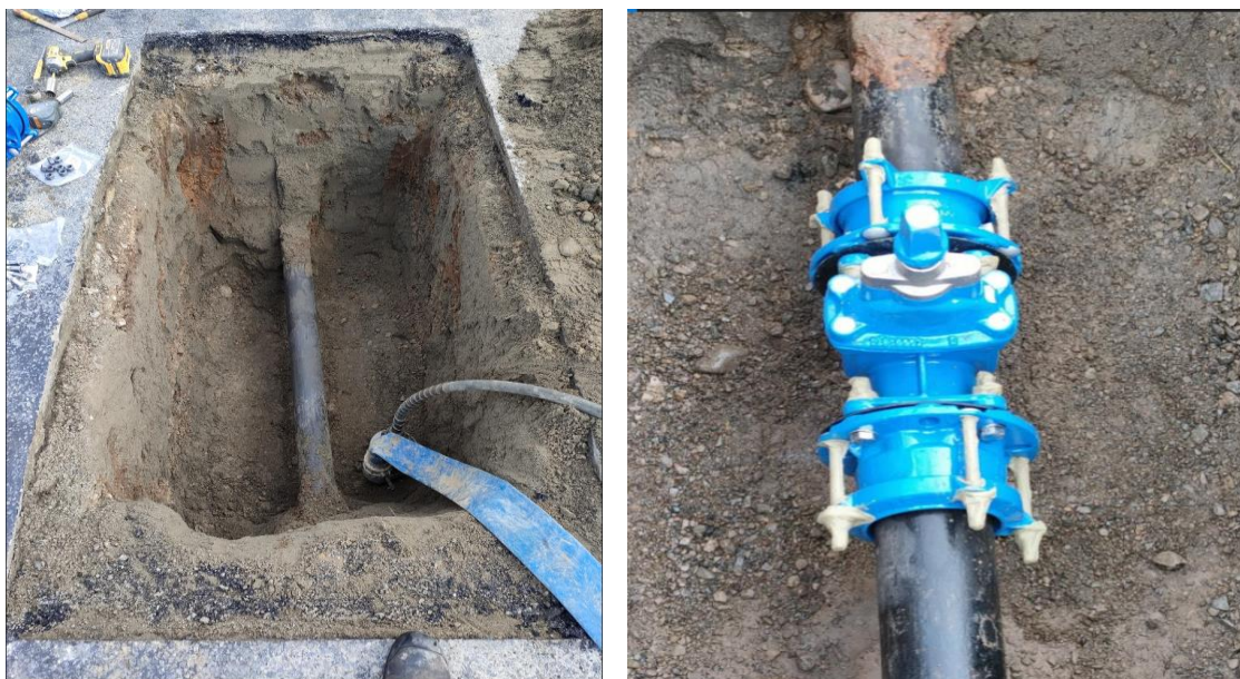
Before (left) and after (right) of a new sluice valve being installed on the Swinburn street watermain
