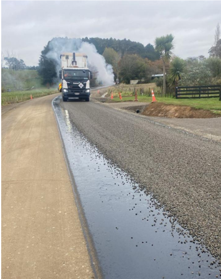
Tararua Alliance rehabilitation team sealing Matamau-Ormondville road.
