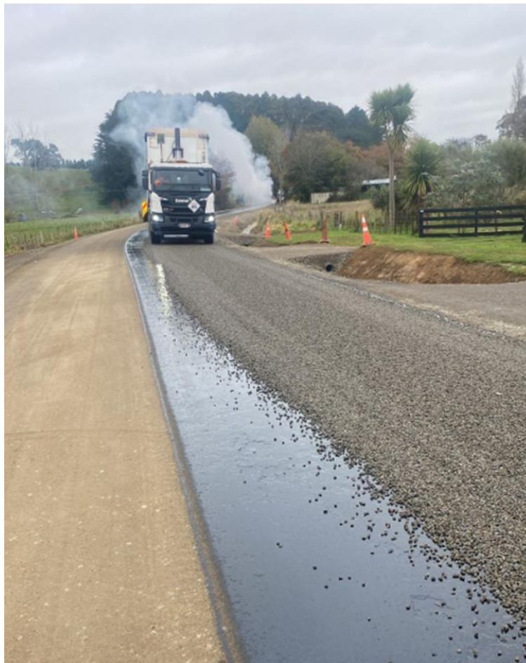
Tararua Alliance rehabilitation team sealing Matamau-Ormondville road.
