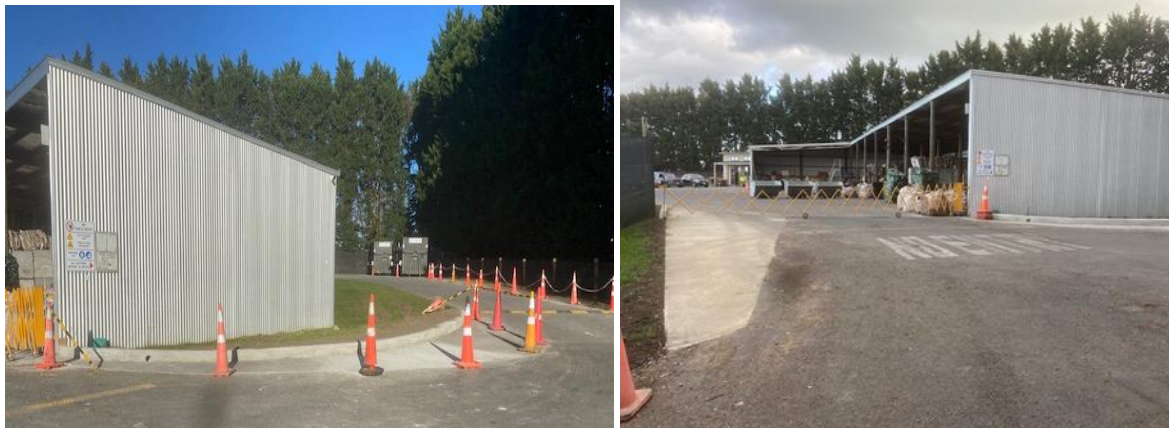
Entrance Way Concrete – Previously muddy puddles in winter
