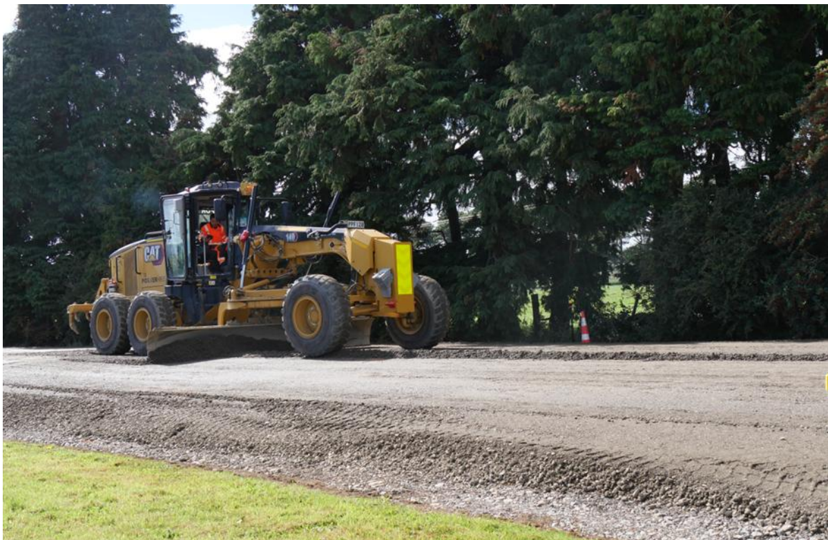
Tararua Alliance Rehabilitation team grading on Top Grass Road.
