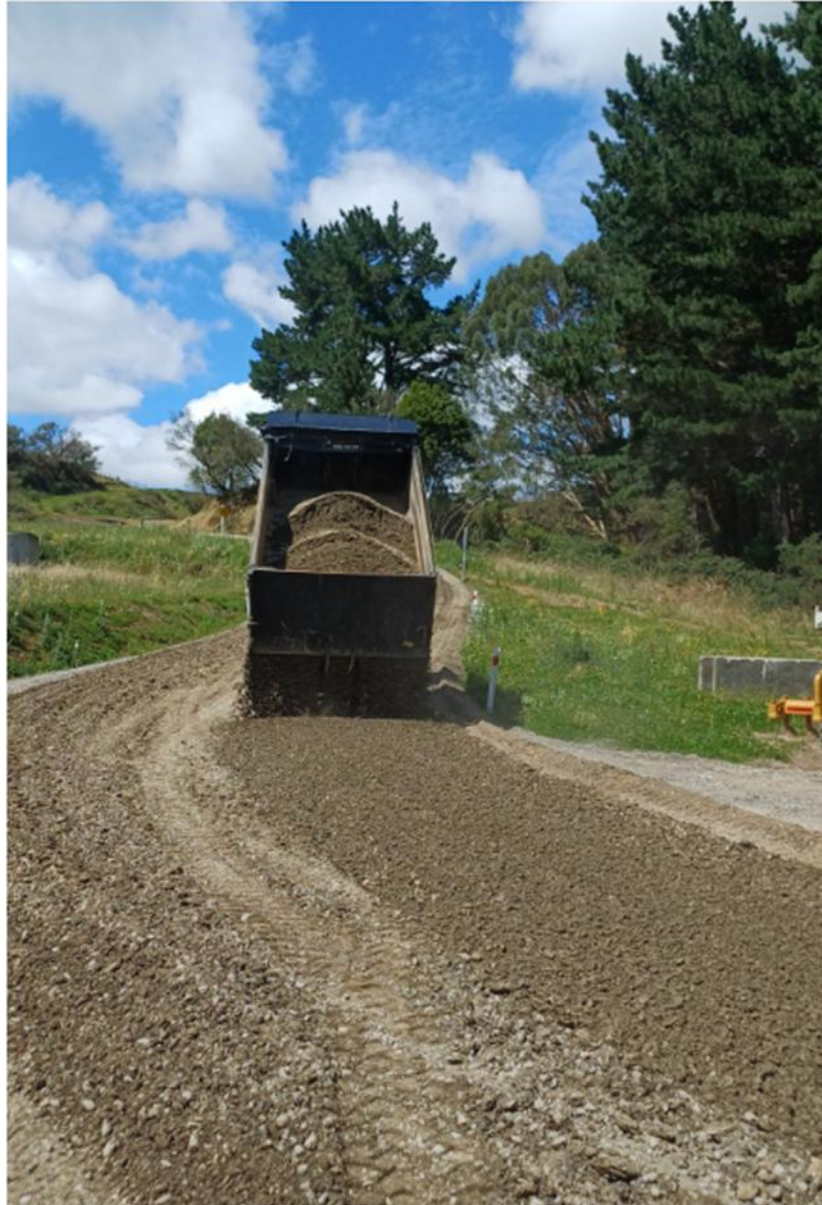
Laying the AP40 ready to prepare the Eastern side for sealing
