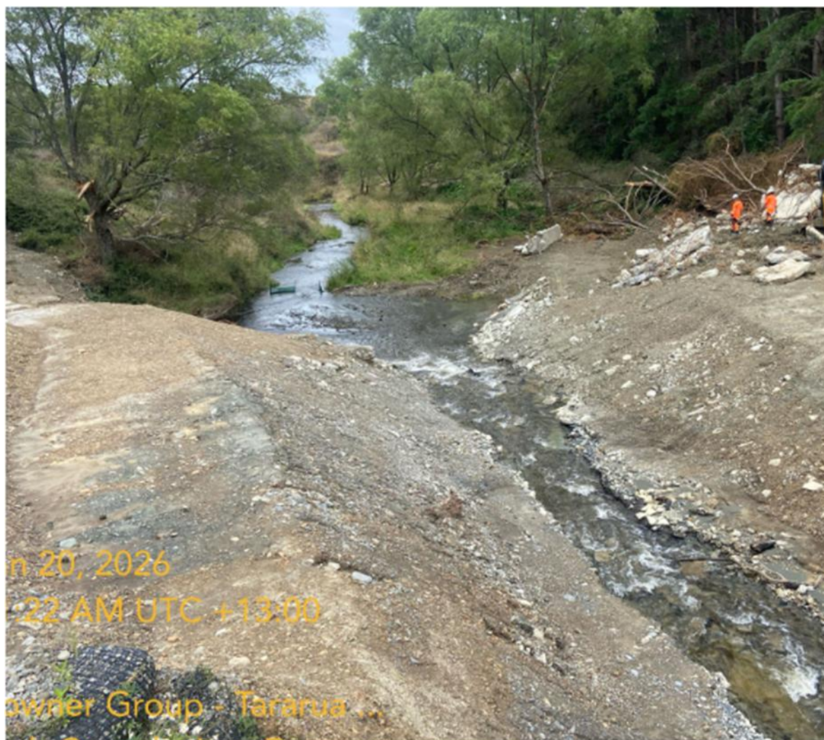
Old box culvert has been removed
