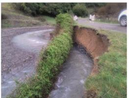
Omata Road, Pahiatua. Erosion is leading to the likelihood of the loss of the approach leading up to a single lane bridge.
