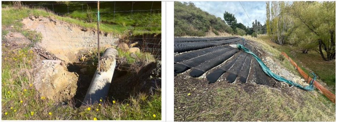
Medium Complexity Culvert outlet repair on Route 52-109.
