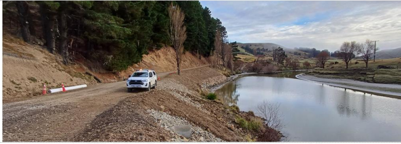
June 2024 – Owahanga Road Rock Revetment and MSE wall nearing completion.
