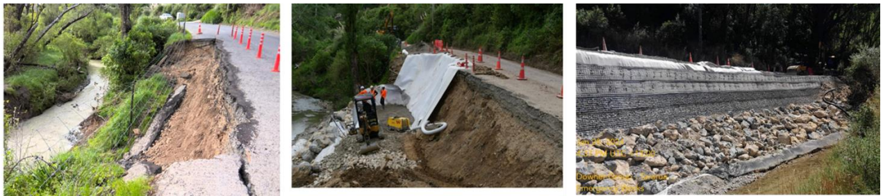
Route 52-63 (RP 3327) – Mass Retaining wall under construction
