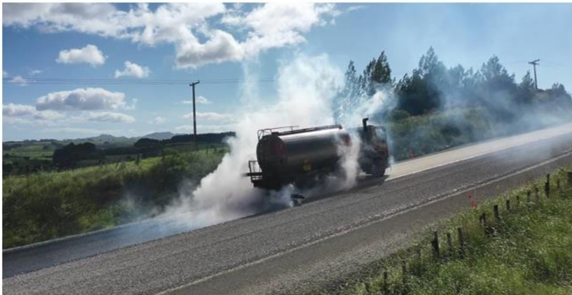
Chipsealing of the Weber Rd rehabilitation site
