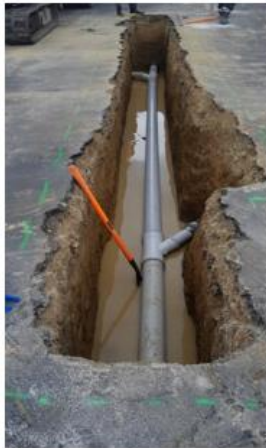
Below Photos – Show a Sewer a Repair in Sneddon St
