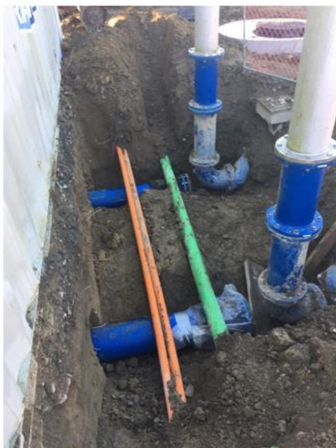
Pipe work thrust underneath existing UV unit
