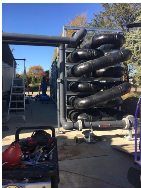
Flocculator assembly
