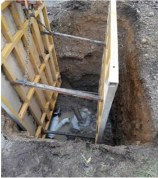
Above photo shows the install of the sewer connection servicing 44 Gladstone St Woodville
