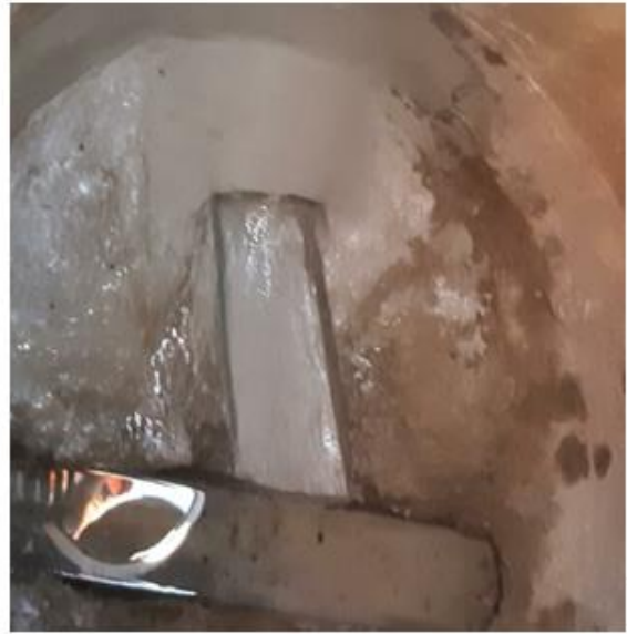
Above photo is showing the new 150mm sewer connection direct to council manhole. This services the 5-section subdivision at 42 Ruahine ST Dannevirke
