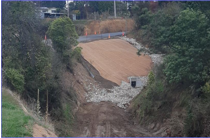
Noreswood / Ormondville Road, Pipe Jacking Project nearing completion
